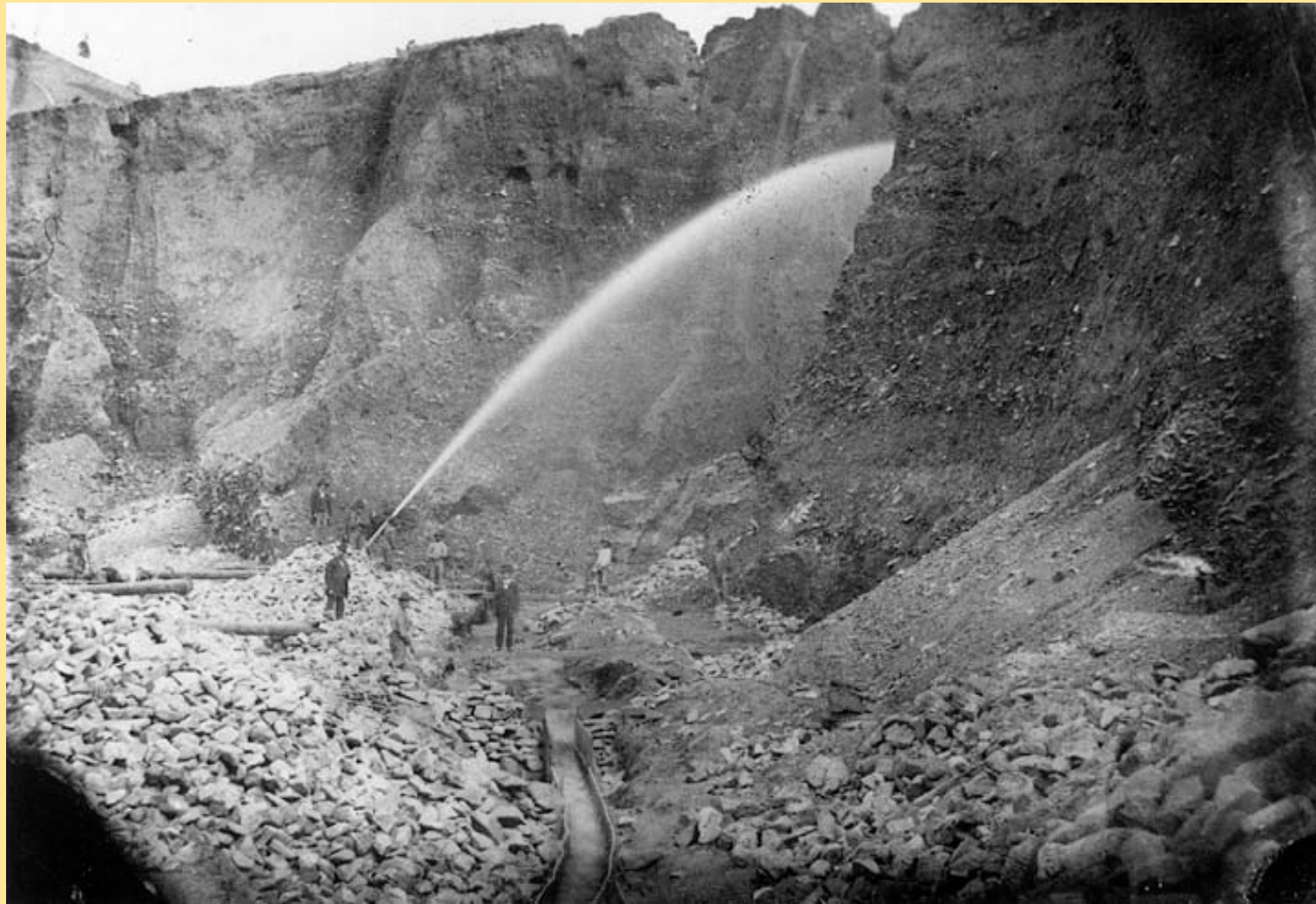
Hydraulic mining at the Lynch Placer in Colfax County, New Mexico, about 1880 (NMBGMR #p-00565)
